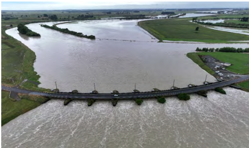
Figure 16: Top: Moutoa floodgates have the highest value of any Horizons asset in the region at $50.8 million in June 2023, and are insured as a part of the Lower Manawatū Scheme. Bottom: Moutoa spillway in operation.
