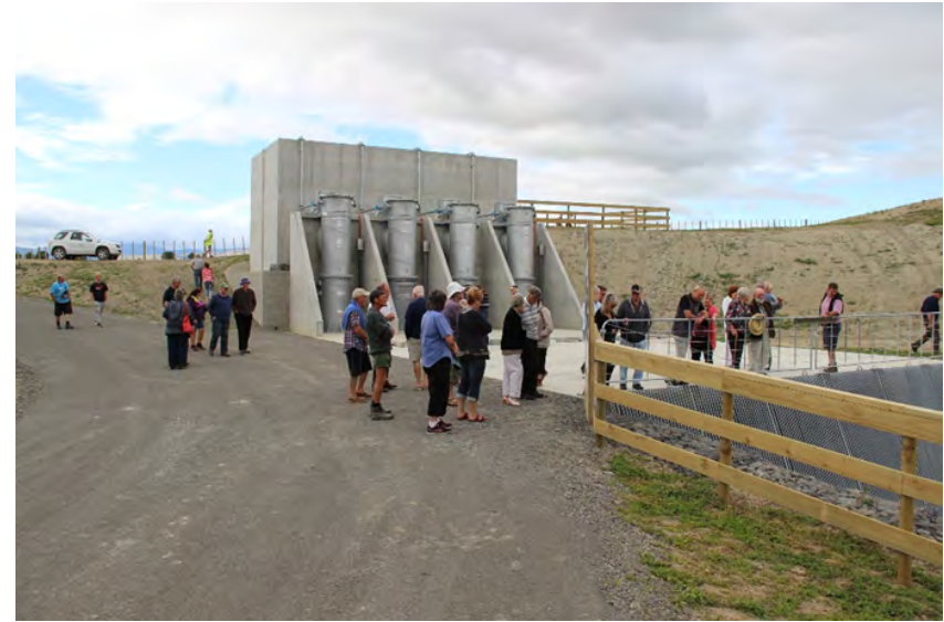
Figure 23: Burkes pump station commissioning/opening 2015. This asset is the biggest of the region's 24 pump stations, and the concrete structure has an estimated life span of 100 years.
