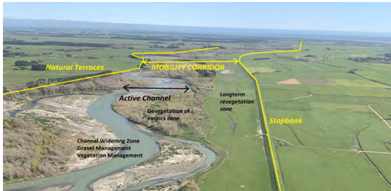
Figure 21: Annotated photo showing the concept of Room for River approach in the Rangitikei River with a mobility corridor, channel widening zone and de-vegetation of exotics zone.
