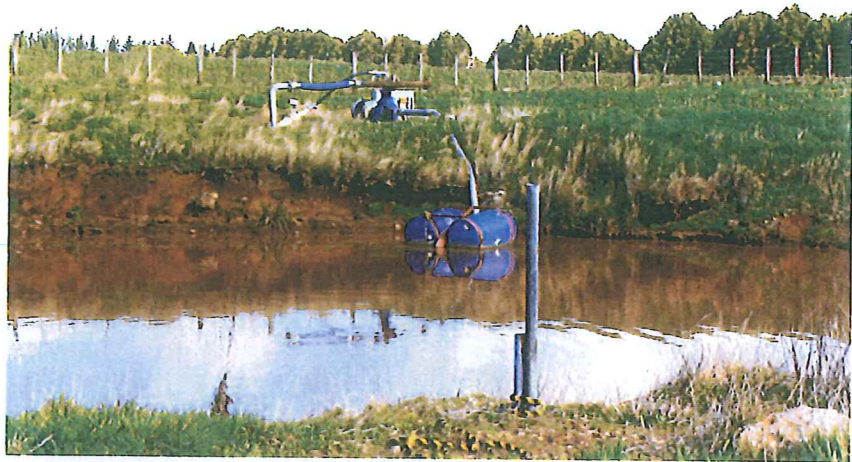
Norman Young, Horopito, pumps water from the last settling pond, which is re-used in the washing plant. Lou Bird
