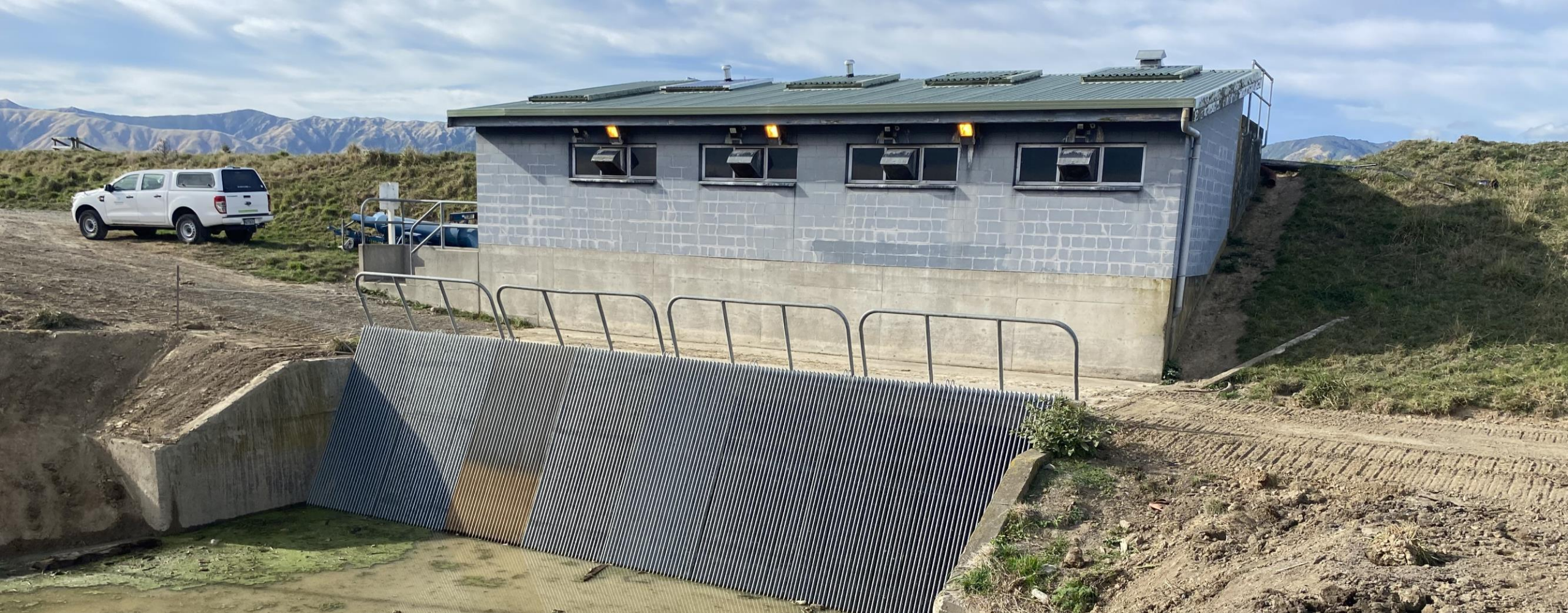
Photo – Okuku pumpstation with grills replaced (April 2024)
