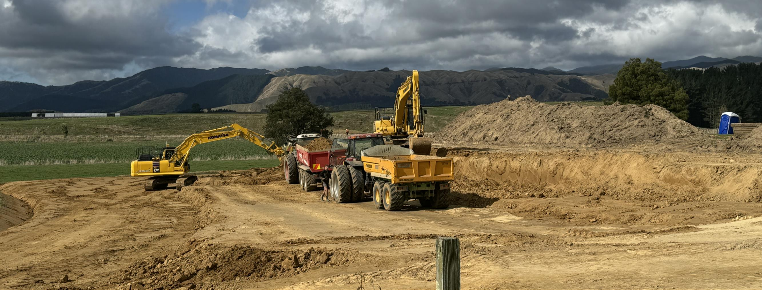
Photo – Koputaroa stopbank refurbishment (April 2024)
