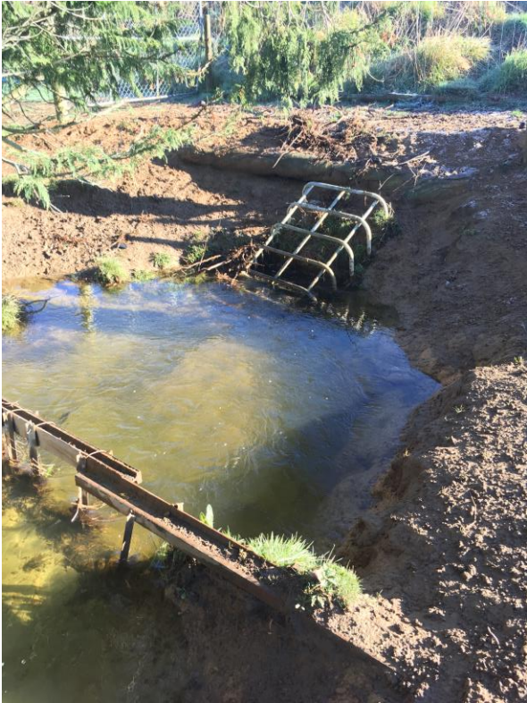
Photo 2: Pakihi Punch Dam inlet
