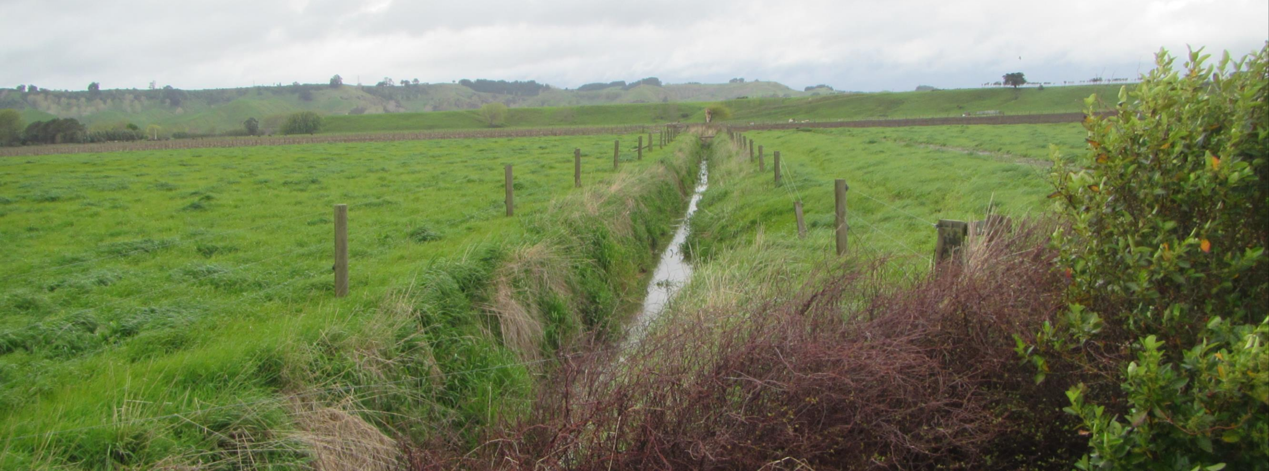
Photo – Haunui open drain
