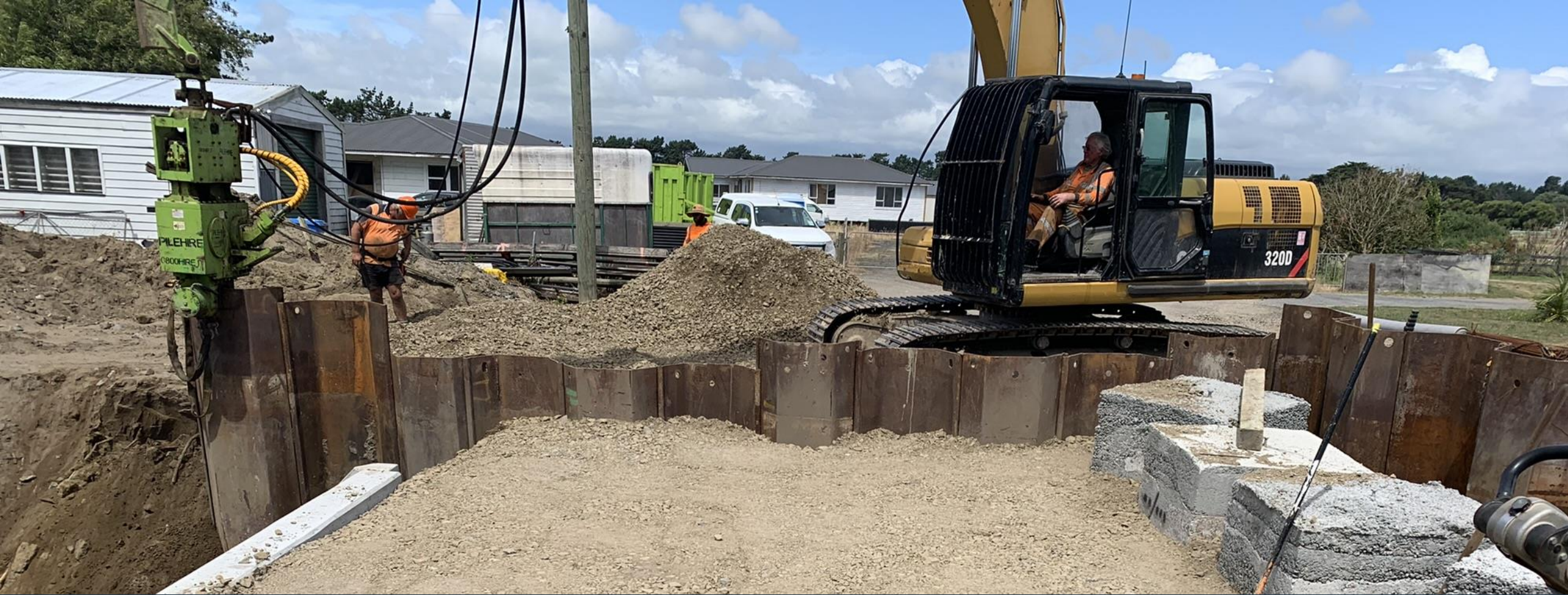
Photo – Upgrade of Coley Street Culvert
