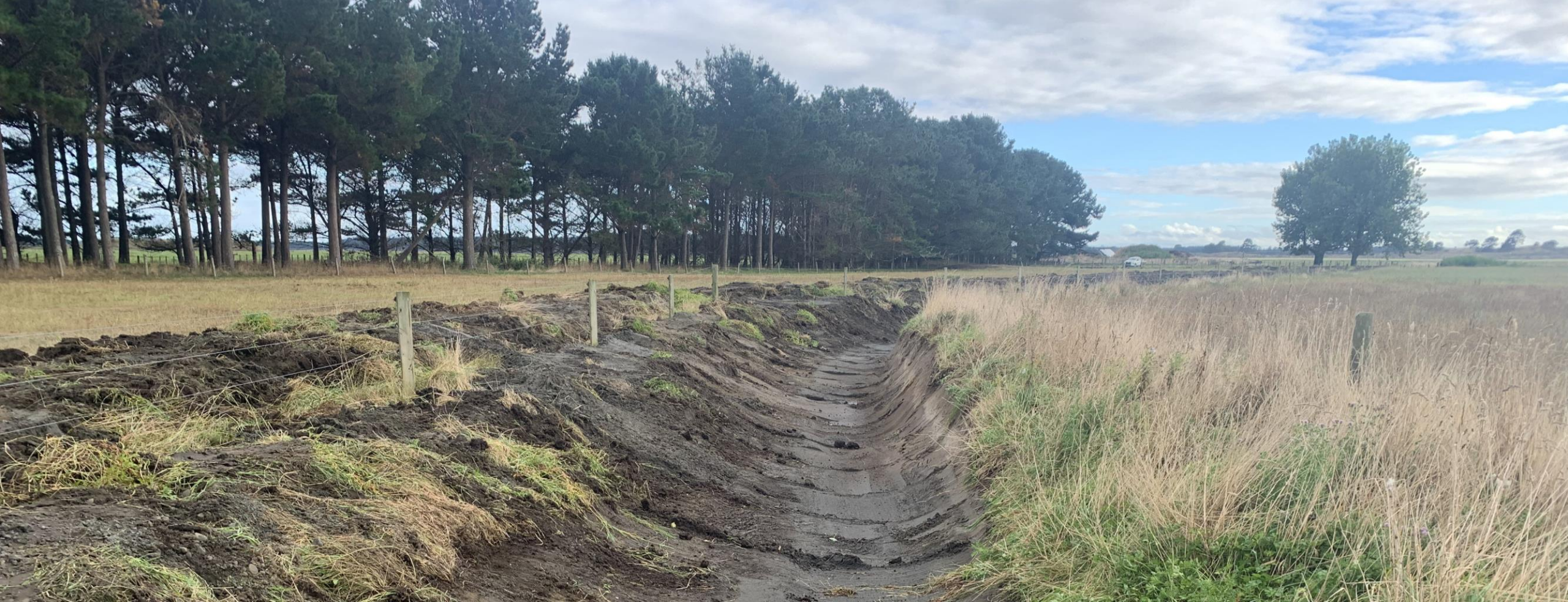
Photo – Forest Road drain cleaning
