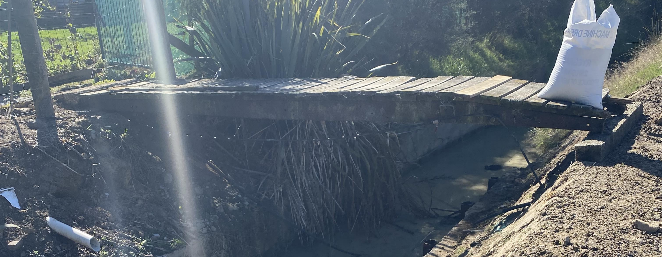
Photo – Asset repair – North Street
