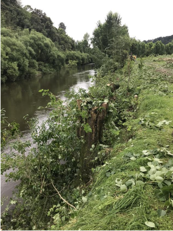
Photo 2: Upper Whanganui Ngahuina (Cherry Grove) vegetation maintenance.
