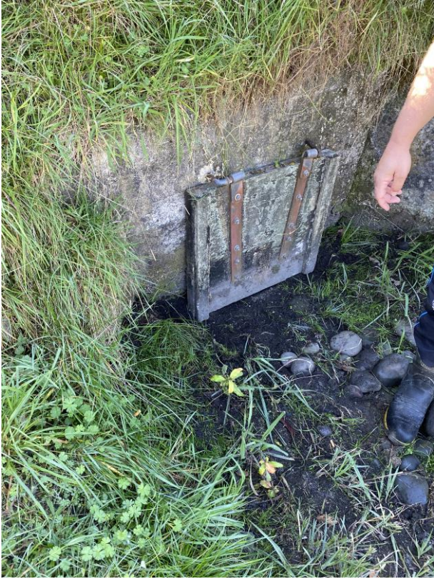
Photo 1: Upper Whanganui Floodgate.
