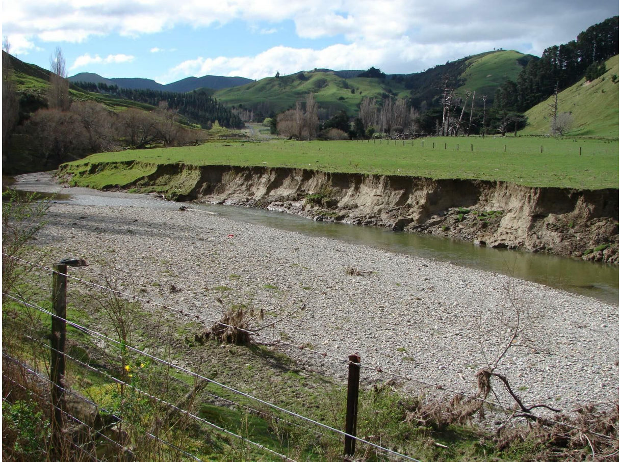
Fresh severe streambank erosion in alluvium near Weber
