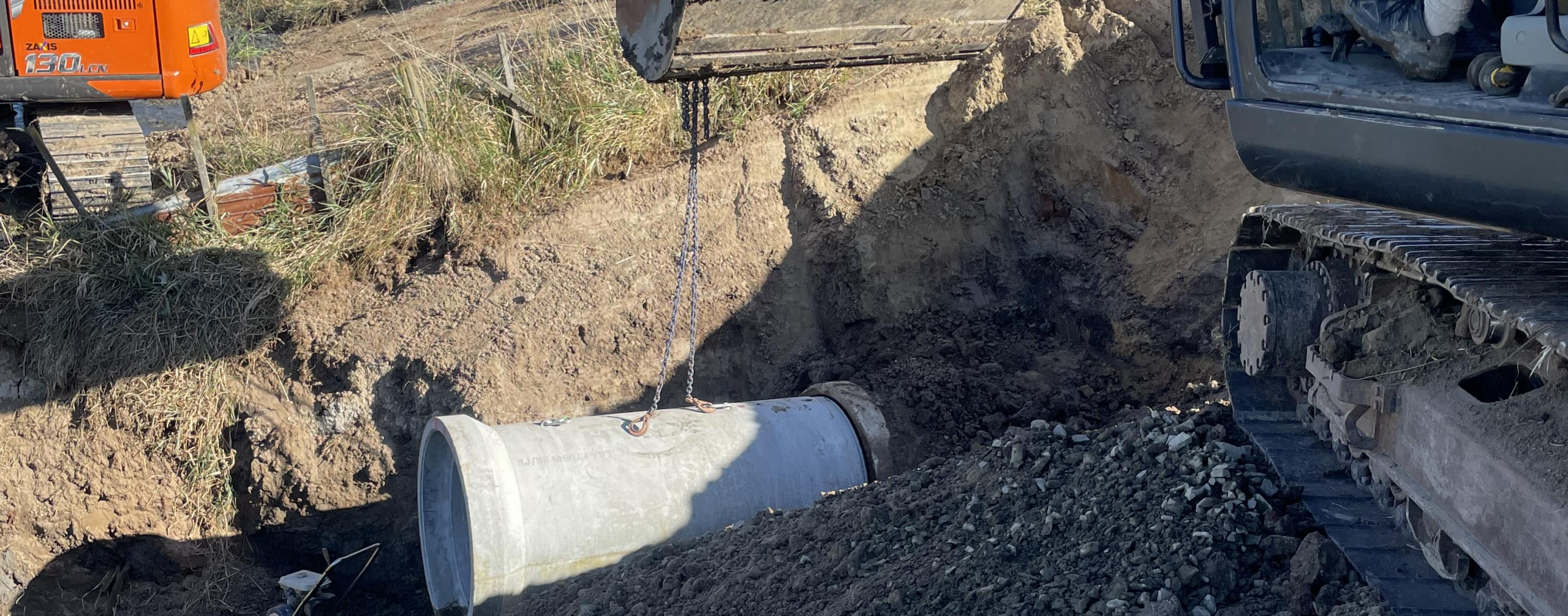
Photo – Culvert extension on Moutoa Spillway
