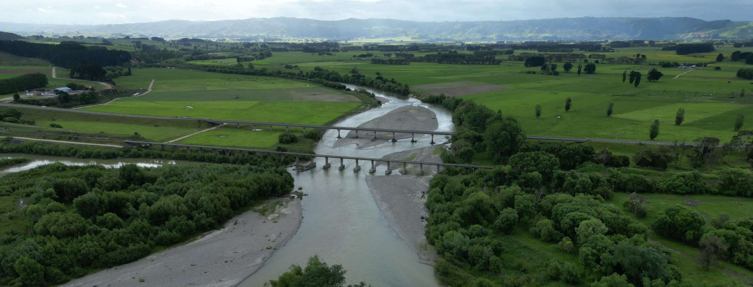
Photo – Tiraumea and Upper Manawatū River Confluence at Ngawaparua Bridge
