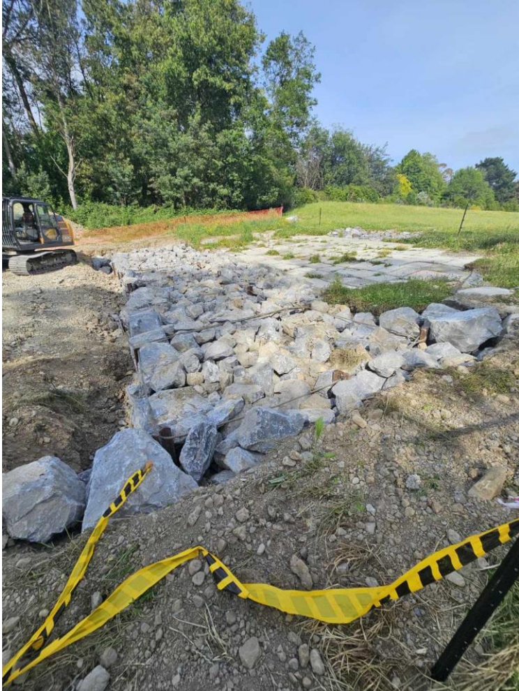
Photo: Makino Spillway outlet
