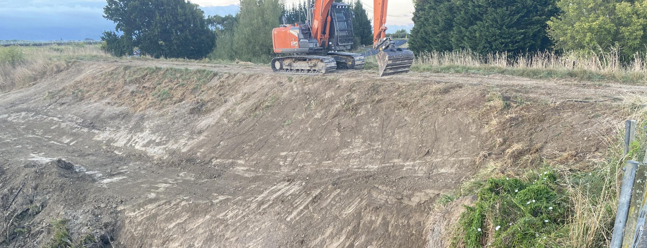
Photo – Repair of slumping at S1 gate outlet
