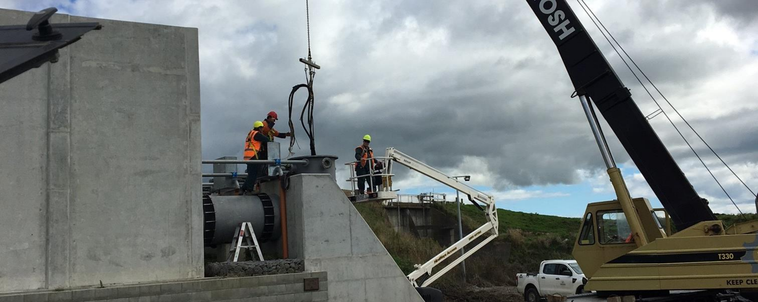
Photo – Pulling of Burkes Pump No. 1
