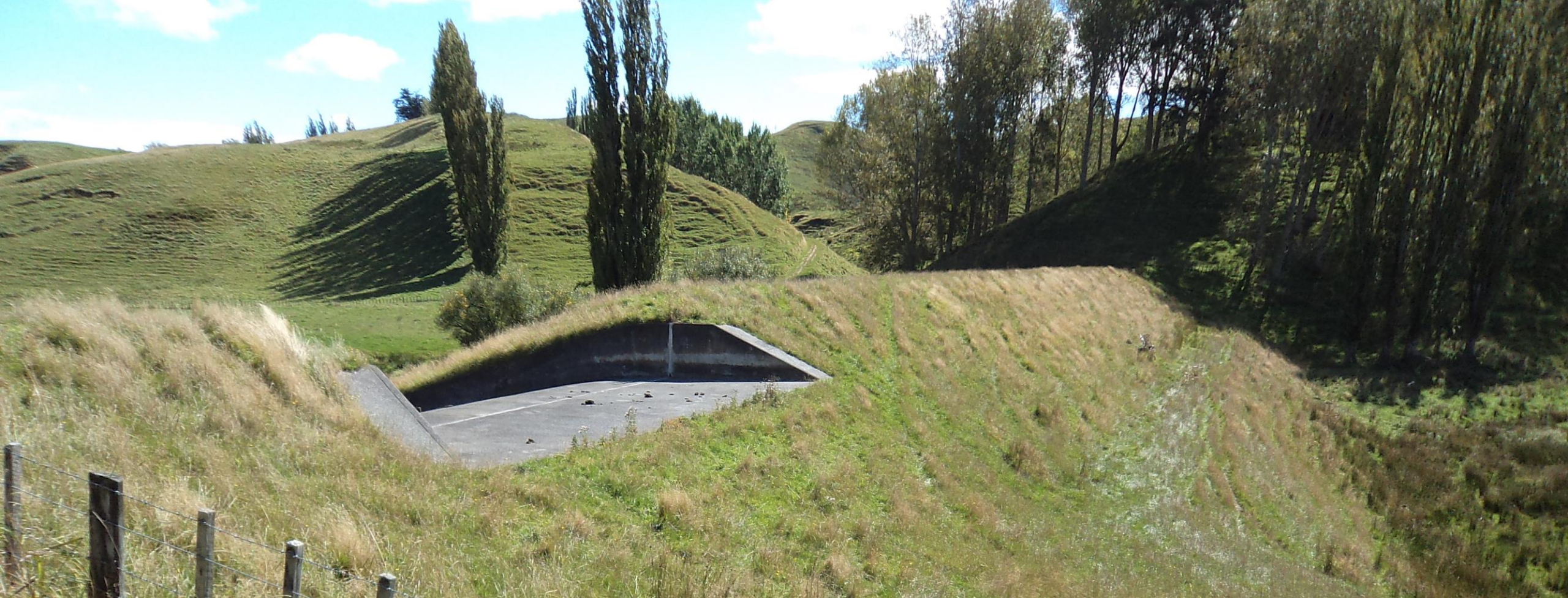
Photo – Detention Dam 46, one of 27 dams in the Porewa Scheme
