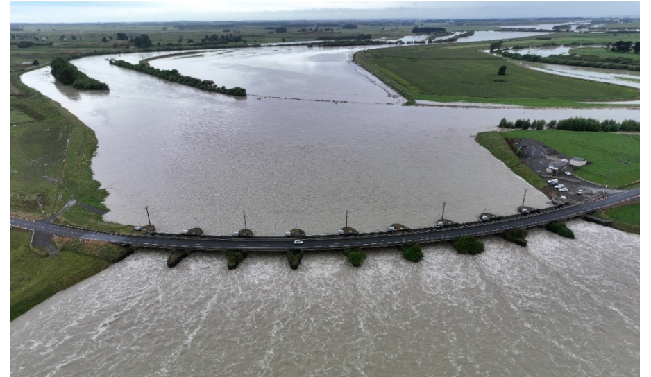
Photos – Moutoa Gates in the Lower Manawatū Scheme.
