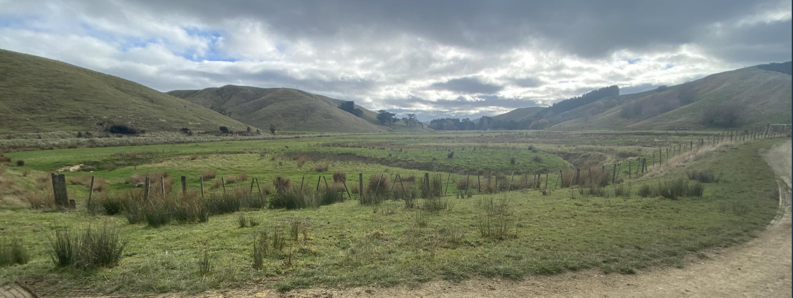
Photo – Tawataia Dam at Spillway Overlooking Tawataia Creek
