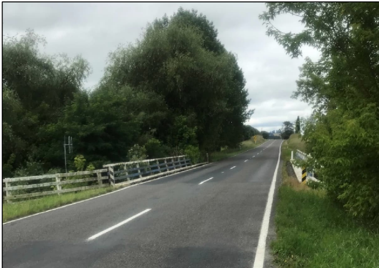
Figure 2.1: Kahahakuri Stream Bridge on Ongaonga Road
